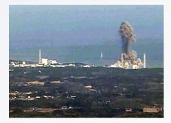
The ignition of hydrogen was the main reason of a blast at a Japanese atomic power reactor in Fukushima in 2011.
